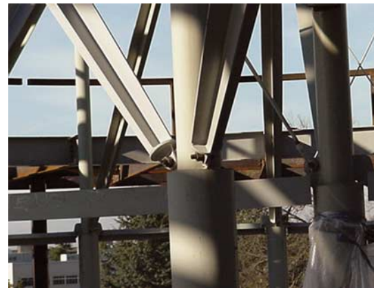
Above, center, and below: The exposed curved roof structure of the central atrium is supported by "tree" columns composed of round HSS "trunks" with "branches" of tapered \frac{3}{8} " plates welded into a cruciform cross-section.
