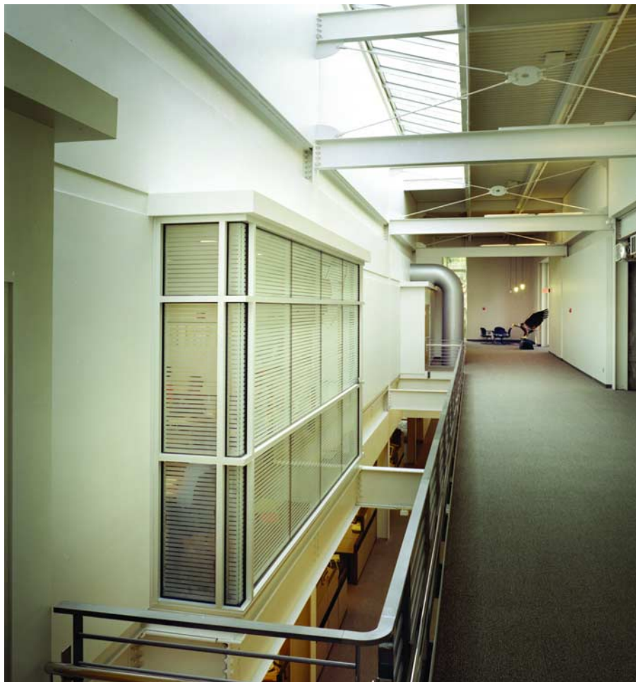
The structure's central light well admits daylight deep into the interior.
