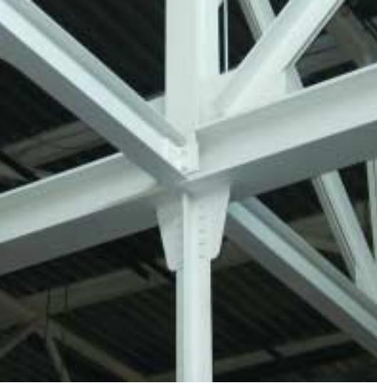
One of the many truss-to-column connections in the Assembly Building. The frame-line trusses and the columns form rigid moment-resisting frames in both principle directions to resist lateral wind and seismic forces. In total, the Assembly Building included more than 1,200 trusses of greater than 350 different types.
