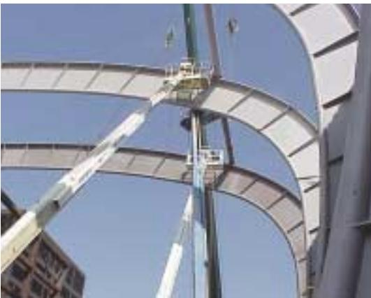
Seventeen curved, steel-bent beam-columns or "ribs" support the roof structure. The ribs were erected in two pieces with a bolted and welded splice connection approximately 60' above grade
