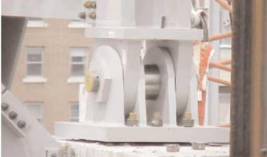
The box trusses connect to each concrete pier with a pin assembly connection.
