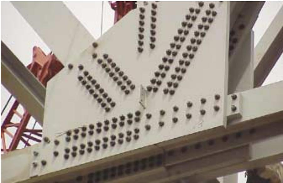
Some of the gusset plates in the box truss are more than 3" thick
