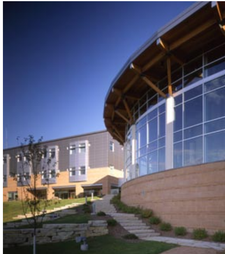
This page: The extensive use of wood framing for the Community Center's roof required that it be structurally isolated from the rest of the hospital to meet fire code requirements. Photos courtesy Hammel, Green and Abrahamson, Inc.
