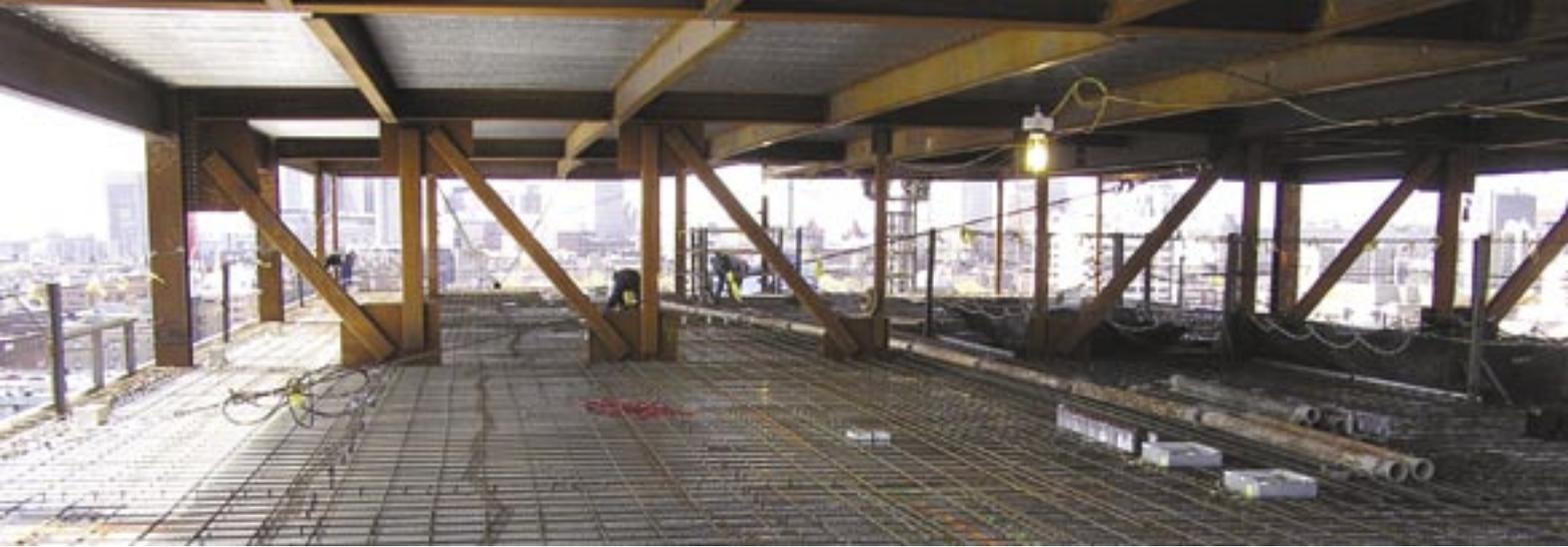
The Macallen Building project features a total of 35 trusses spaced at 36 ft o.c. and spanning 64 ft, 4 in.
