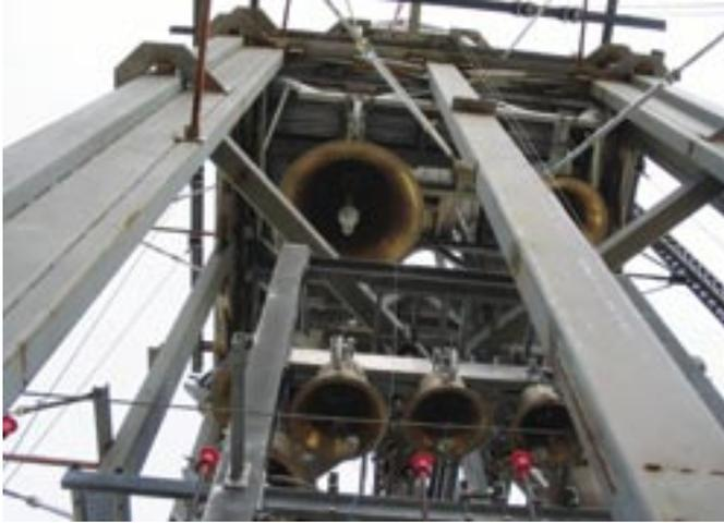
The structural steel framing supports a 50,000 lb, 49-bell carillon in addition to a 14,000 lb pre-manufactured steeple.
