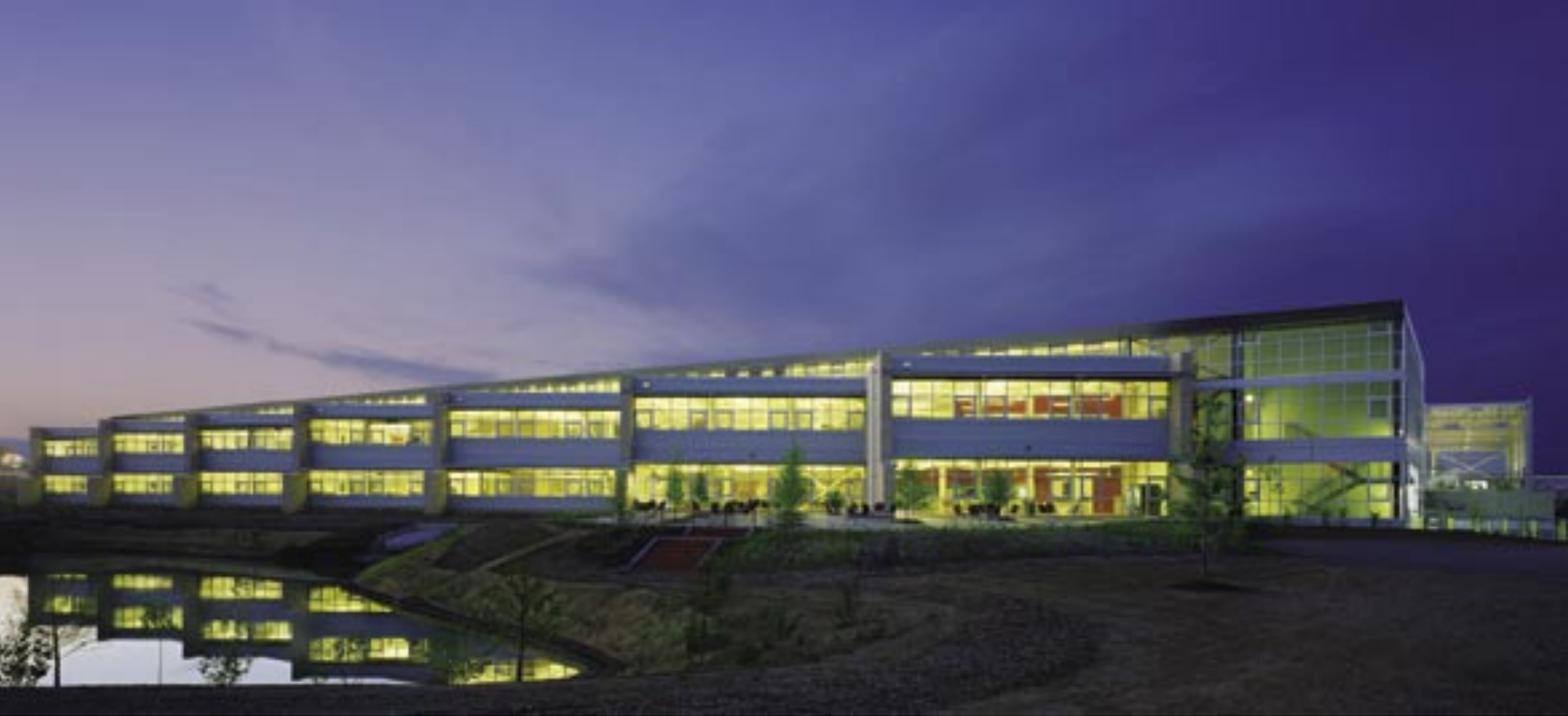
The steel-framed “saw tooth” design of the exterior walls was created to reorient the building, which had faced southwest, to essentially face south. This allows more daylight into the office spaces while providing relief from direct afternoon sun.
