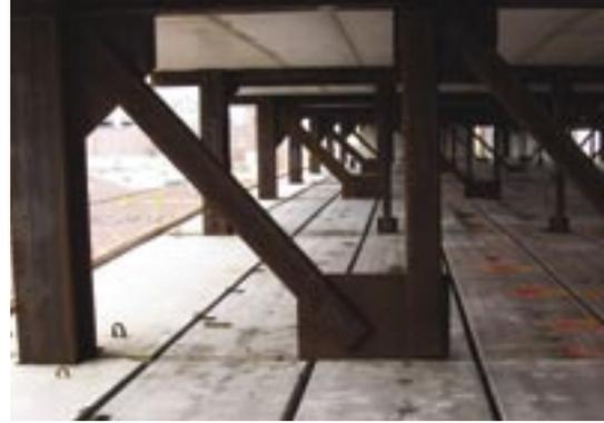
Staggered trusses were framed into the walls between hotel rooms. Floors are framed with 4-ft-wide, 10-in.-thick precast prestressed concrete planks. The planks span 30 ft between the bottom chord of one staggered truss and the top chord of the next.
