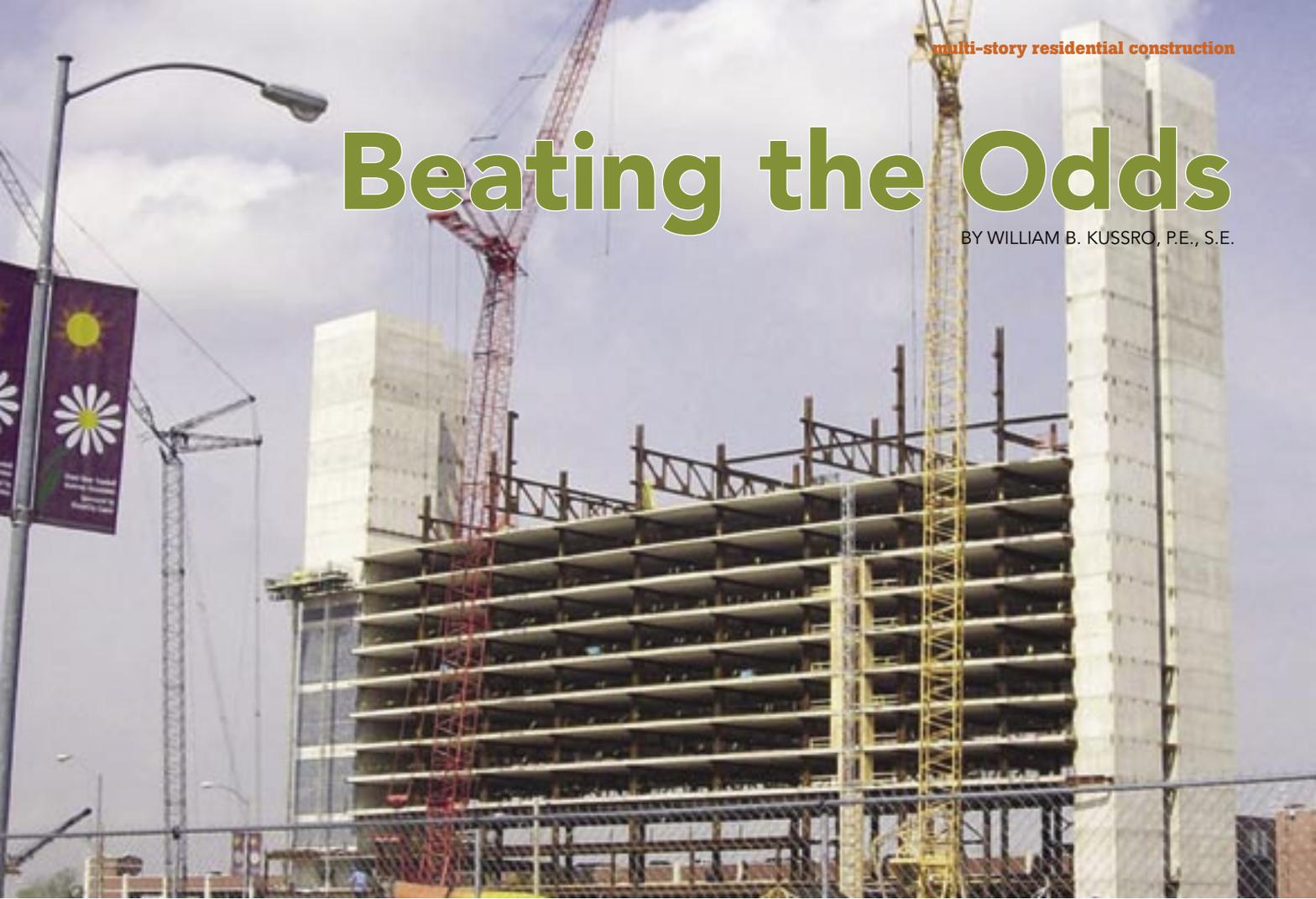
**Staggered steel truss framing makes this Detroit casino/hotel a winner, while maintaining both the floor-to-floor and overall structure heights of the original concrete frame design.**
