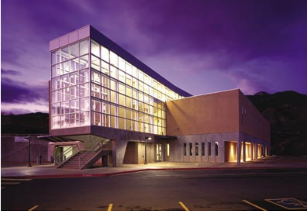
One entry features a glass and steel “tunnel” framed with HSS 10x6 members.
