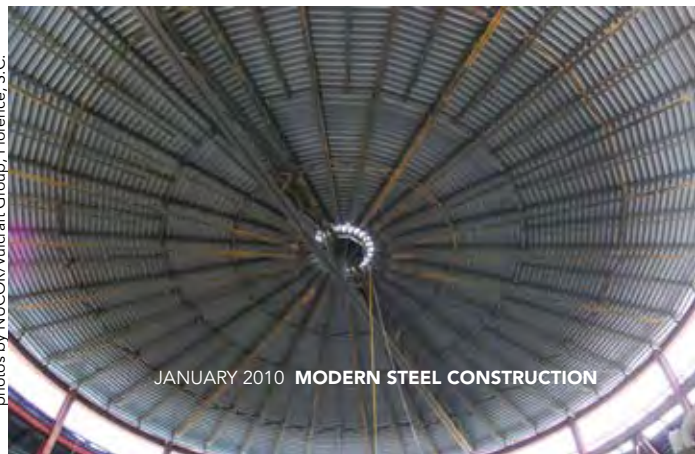
Below: Half-length joists on the lower portion of the slope between the full-length joists reduce the maximum metal decking span. The upper ends of the half-length joists are supported by an intermediate header.
