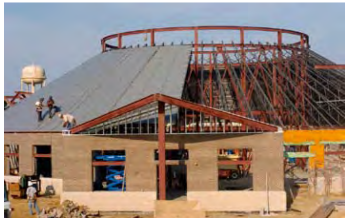
Above: Placement of steel decking to form the roof of the office complex followed quickly after the sloping joists were put in place.
